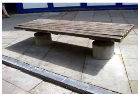
Typical timber bench in need of repair
