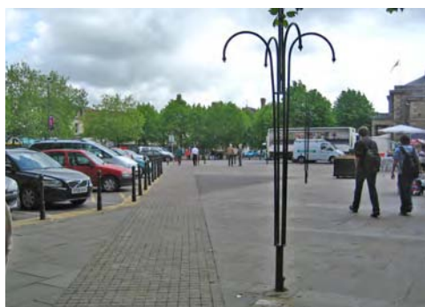
Yorkstone paving and redundant hanging basket post
